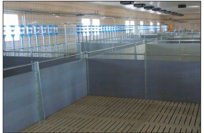
the system of PVC profiles fencing in the gestation sector
